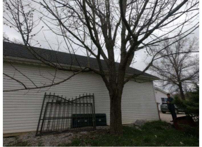
Tree may be rather close to home and cause issues with gutters roof and foundations.
