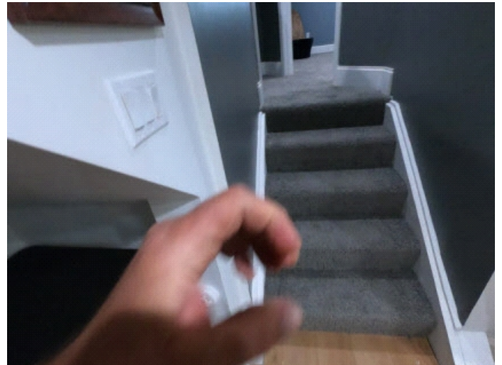
Missing handrails.
