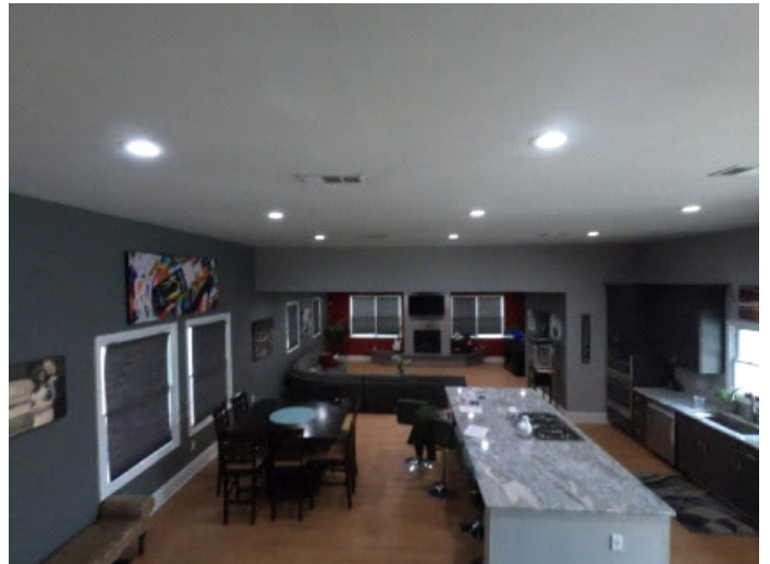
Sometimes can't recessed lights or ceiling penetrations contribute to heat loss to the unconditioned attic space. This can create or contribute to winter ice dams.
