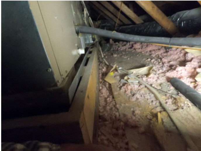
Attic partially floored.
