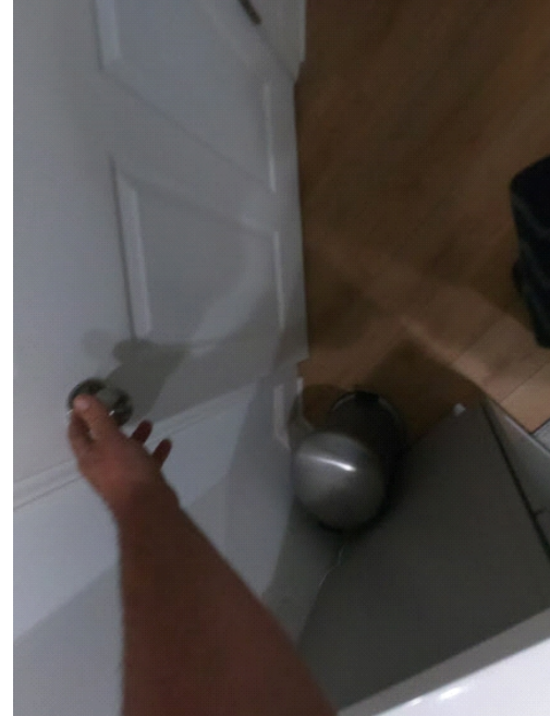
Doors were functional. Some doors may need adjustments.
