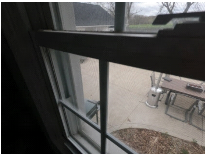
Most screens intact.
