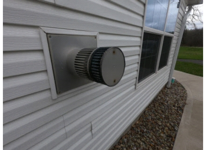
Gas fireplace need to be inspected tested and certified prior to use.
