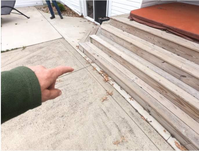
Hot tub was off and not tested. Recommend hot tub company to energize, clean, adjust or perform maintenance. Home inspector did energize and did not inspect the hot tub.
