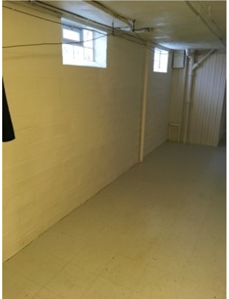
Foundation walls have been recently painted
