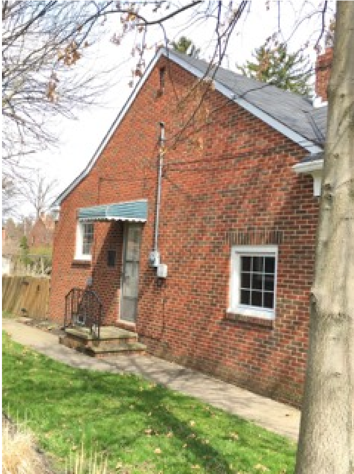
West side of the home.
