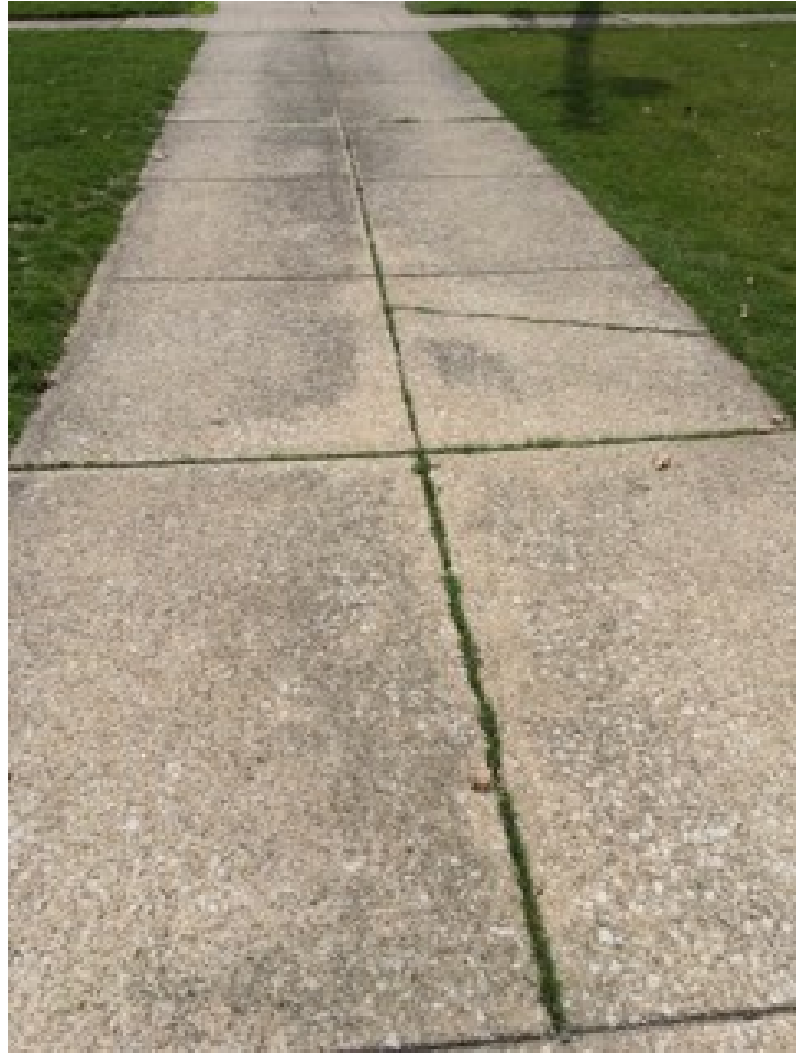
Single car concrete driveway
