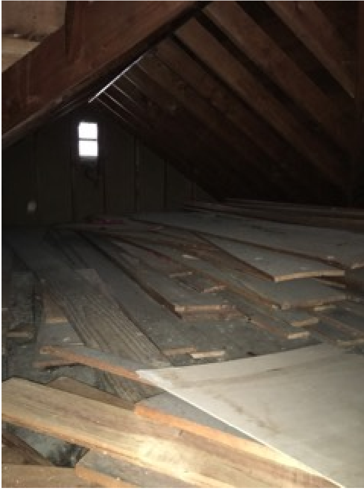
Attic floorboards were removed for the insulation.
