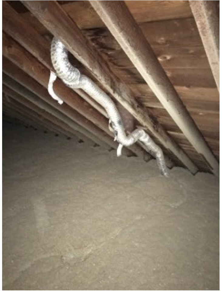
Straighten the bathroom exhaust vent pipe.
